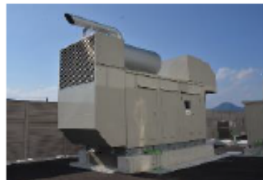
Large Emergency Power Generator with 72-hour Capability
